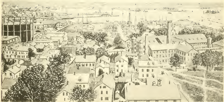
VIEW FROM RHODE ISLAND HOSPITAL
